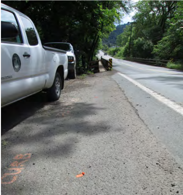
Pedestrian Bridge prior to replacement
