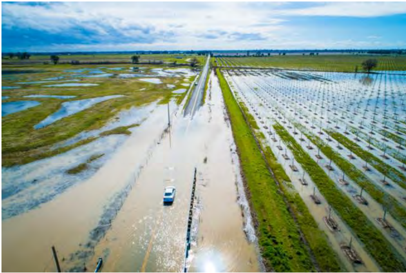
West County flooded road during 2023-2024 winter storms
