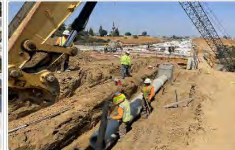
Item # 85, Cal Valley installing D.S. # 1 18" PCP
