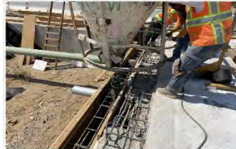
Item # 70, MCM pouring abutment #1 backwall/PT blockout
