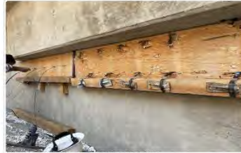
Item # 2, MCM stripping the bridge abutment habitat
