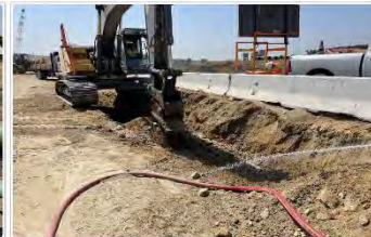
Item # 111, MJD back-filling the 16" watermain north of the bridge.
