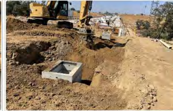
Item # 74, Cal Valley installing D.S. # 1 DI's
