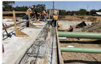
Item # 70, pouring the abutment #1 backwall/PT blockouts
